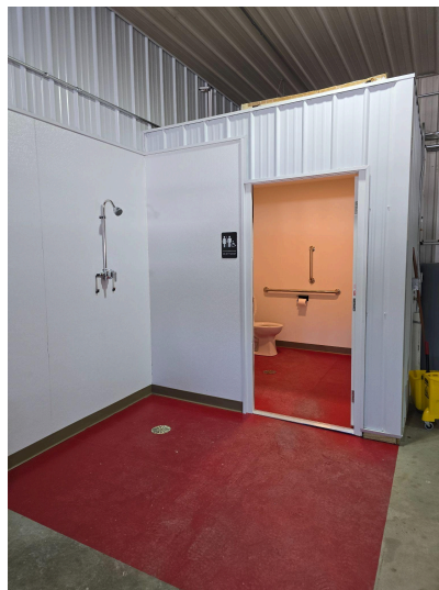
New bathroom and decontamination area
