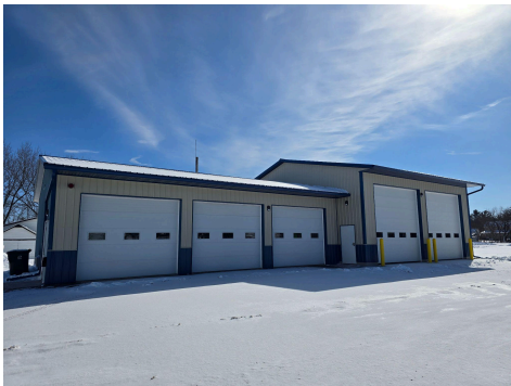
Department After Addition
