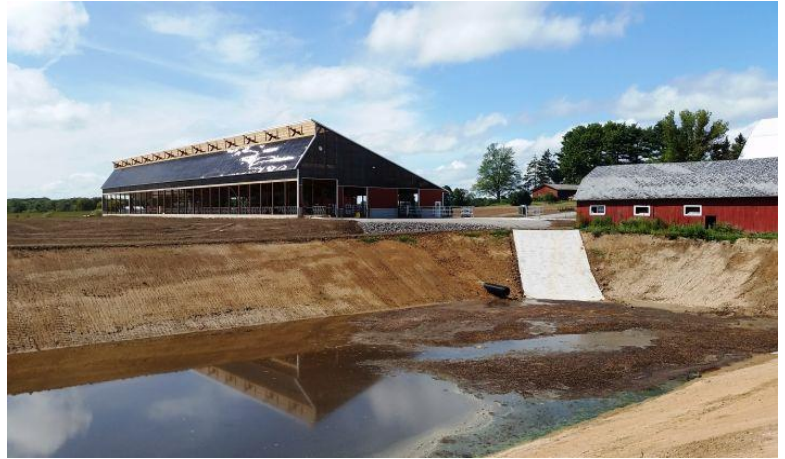
Clay lined waste storage facility
