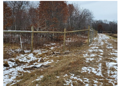
BudzNBudz Cranberry Wildlife fence build
